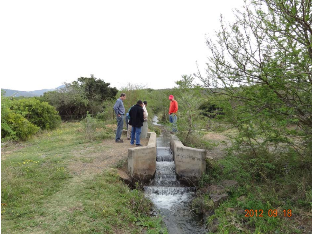
Photo 14 Outlet of canal at point of discharge to Adelaide Municipal Dam
