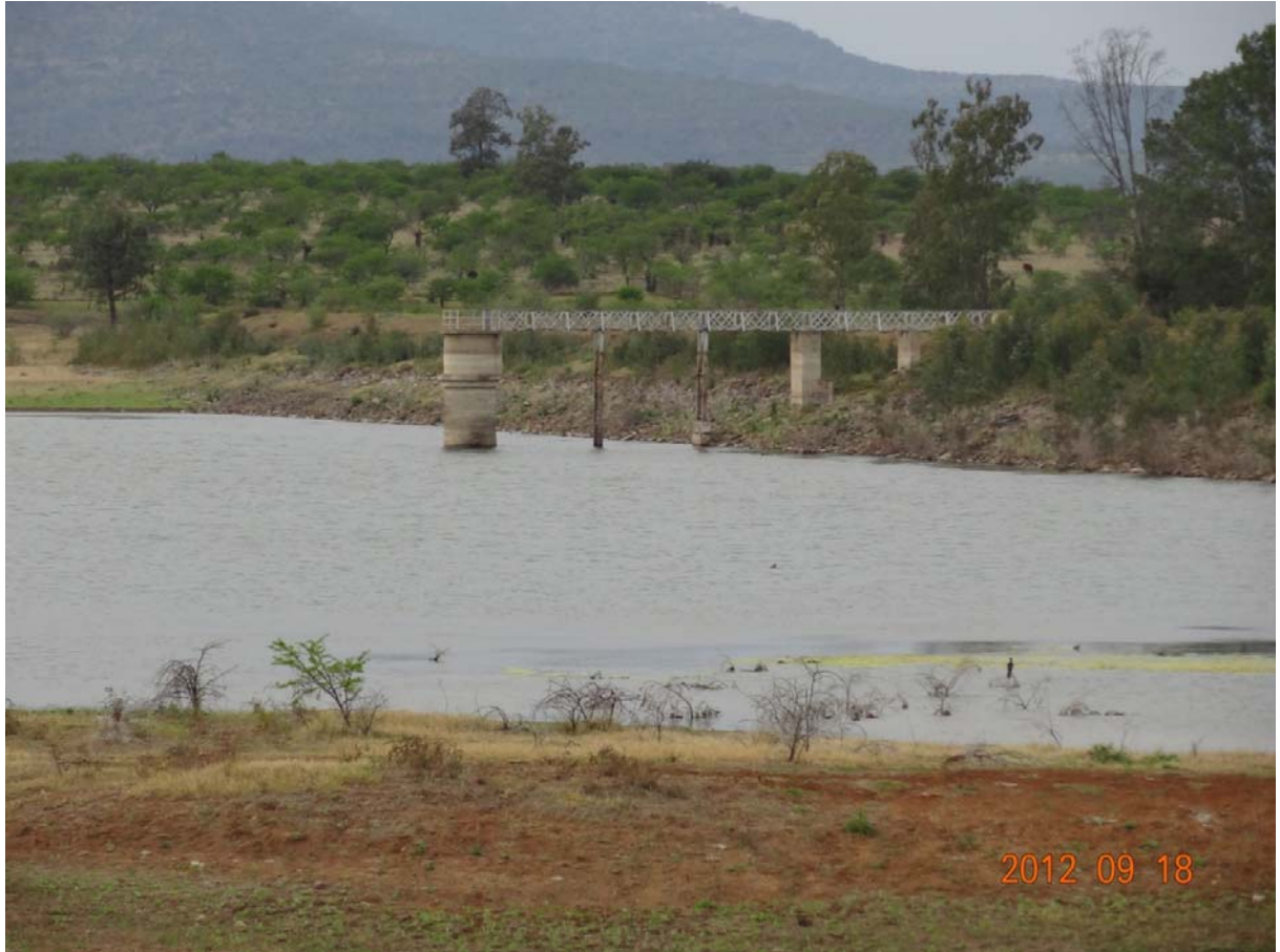
Photo 16 Extraction column within Adelaide Municipal Dam, supplying water treatment works
